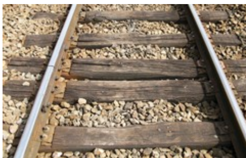
Figure 12: Rails courts sur traverses bois
